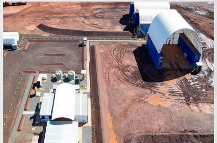
Christmas Creek Fuel Farm Facility
